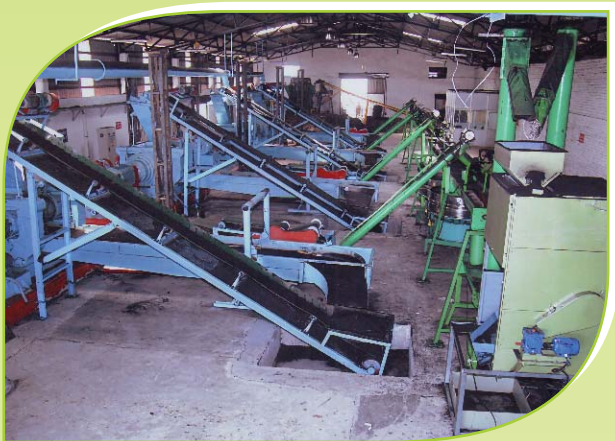
Rubber Crumbing Plant
